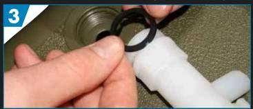
Position seal so that the outer edge with blue marker now sits against ridge facing away from tap thread.
